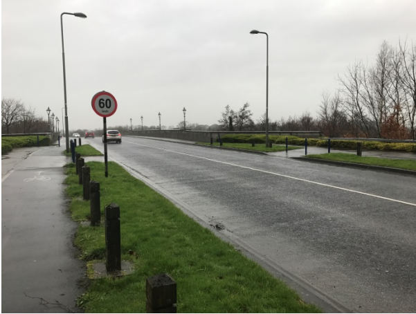
Figure 4: Uncontrolled crossing (typical of local area)
