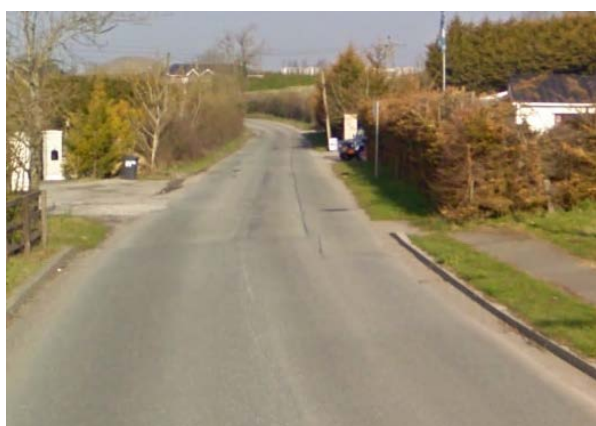
Figure 2: Existing Kerdiffstown Road (looking north-west), showing footpath cessation to the right.
